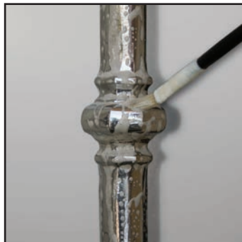
Application of the de-rusting product E4052/D: all polluted parts must be covered
